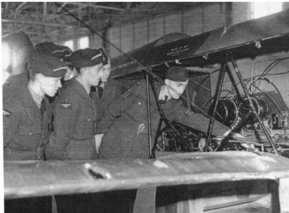
Air frames and Instruments formed an important part of the course and this Group was here being introduced to “GEORGE” the important automatic pilot that the Skipper could, at his decision, to utilize.CH.12472
