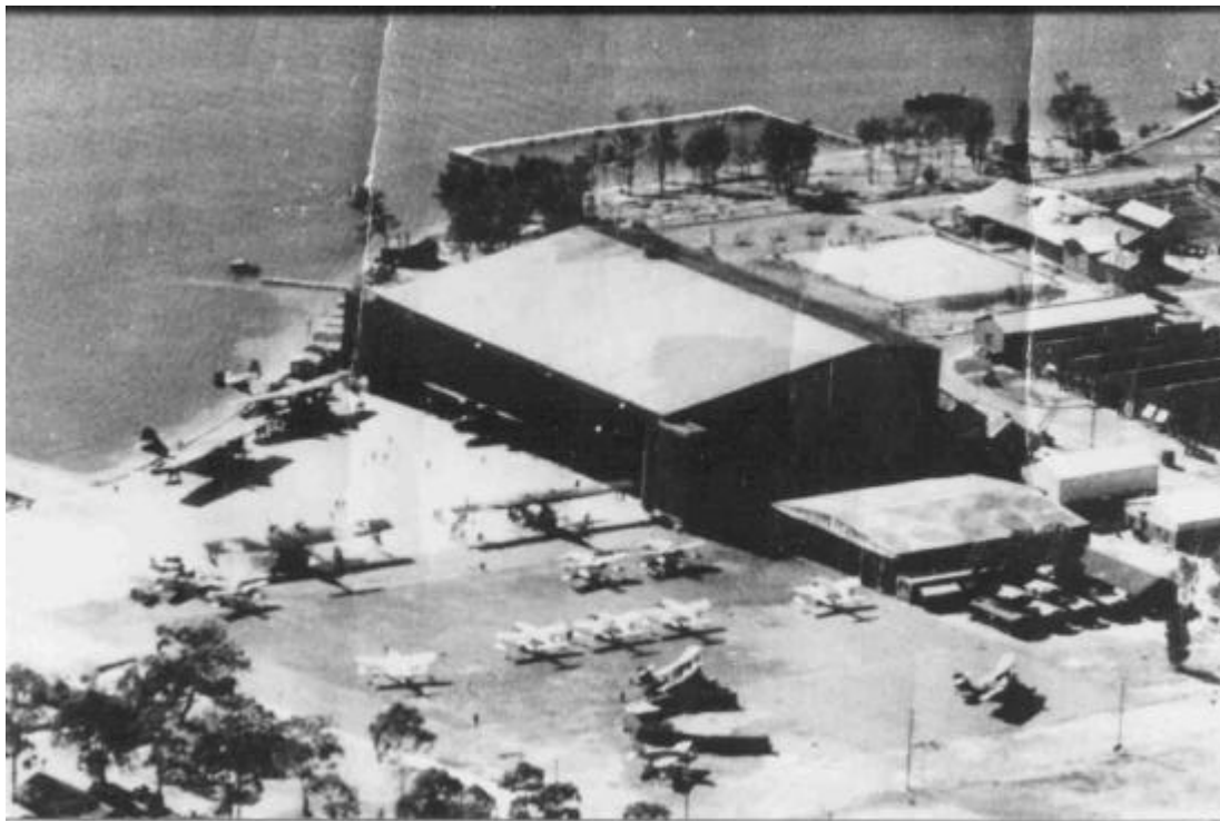
A variety of Flying Boats & Sea Planes are undergoing servicing and maintenance in the hangars and on the hard stand.
