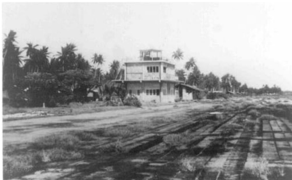
The war time steel mesh runway, with weeds & shrubs appearing, was initially a major problem. It had to be torn up and discarded off shore before work could commence on the new international Air Port. (Point Cook Museum)
