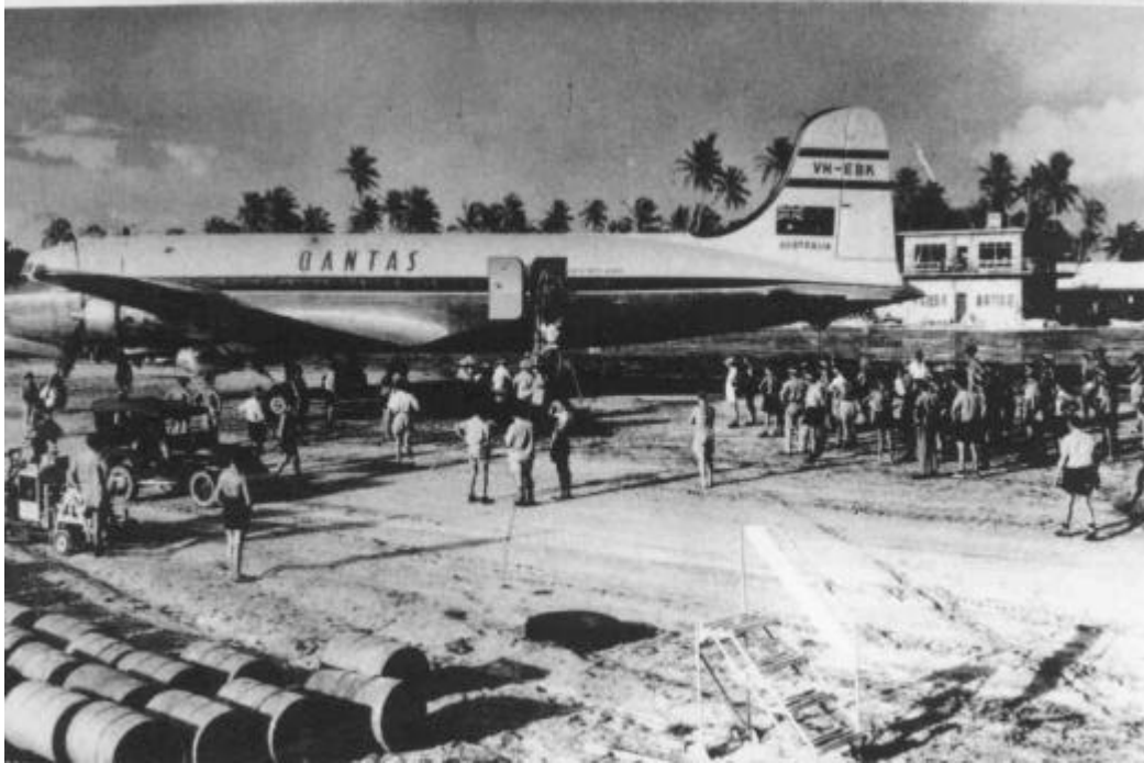
During construction of the airfield, QANTAS Courier aircraft regularly brought in fresh foods and RAAF personnel. (Mrs Sella Lings)
