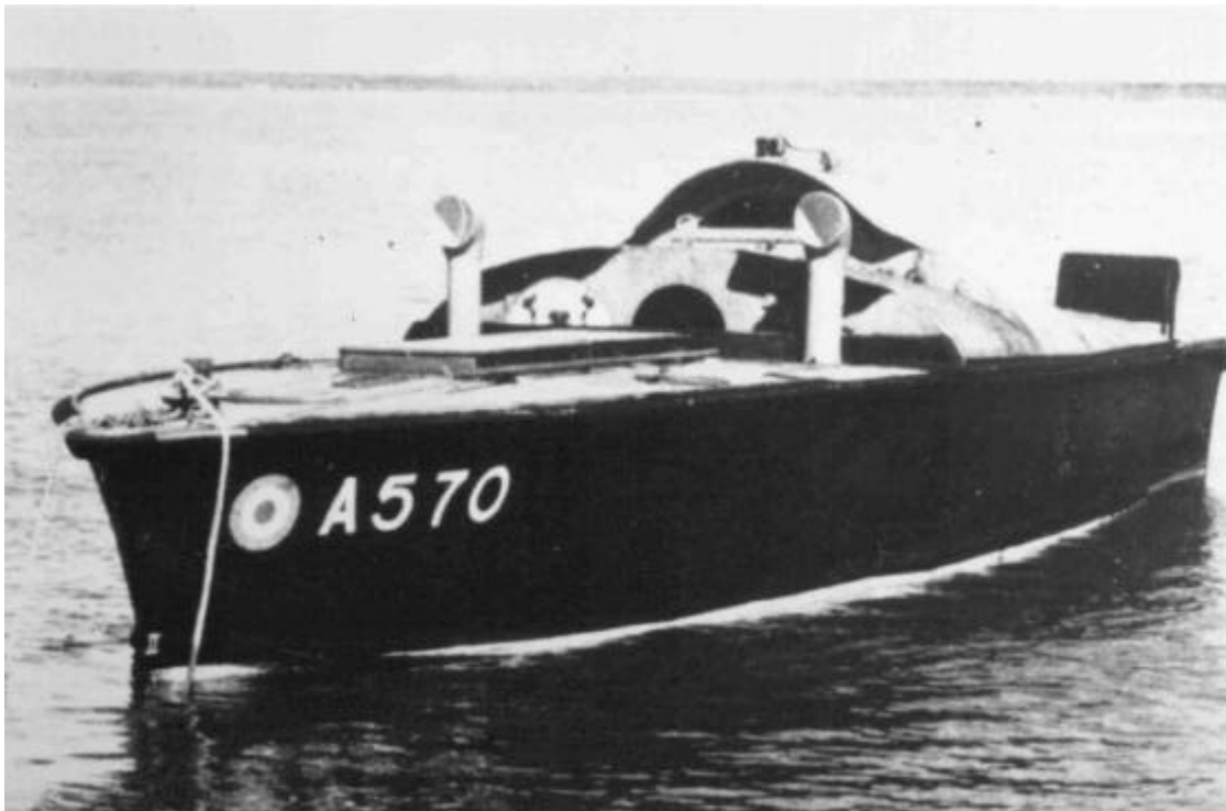
The steel plating on the Target Boat made it top heavy so PLTOFF Bill Lucas applied to have it removed then operated with the target being towed.
