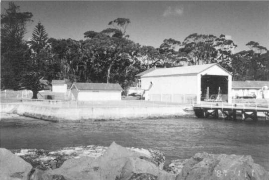
The current facilities still operate at Jervis Bay.
