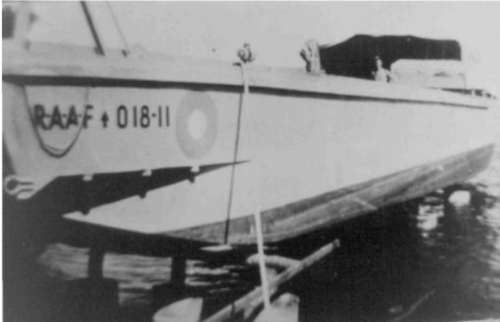
To anti foul 018.11 Landing Barge the Marine Section constructed this device so that when the tide went out servicing & painting could be undertaken. (Gordon Sharwin)
