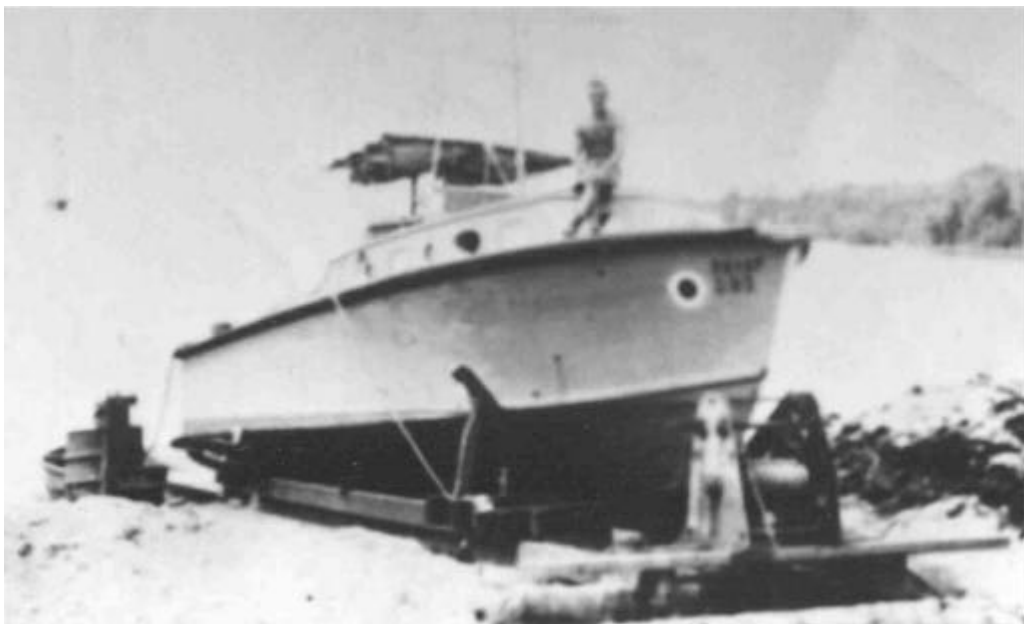
Jack Couch constructed this slip way from scrap taken from a sunken ship and the timber from coconut palms. Maintenance and painting could be more effectively carried out. (J.Couch)
