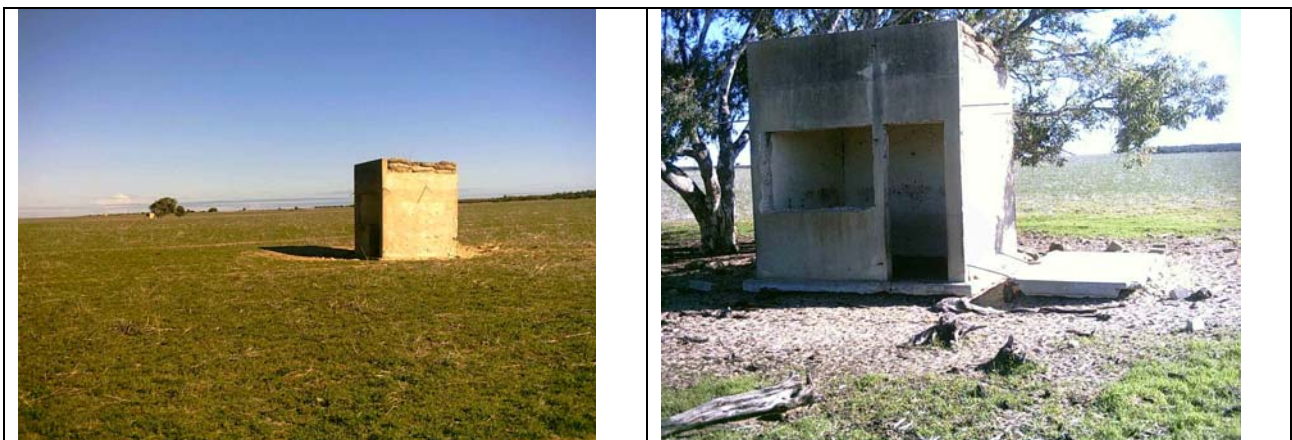
There are three concrete Pill Boxes located away from the bombing target was where Armourers took shelter when plotting sightings where every practice bomb landed. This larger Pill Box, located between the other two, was where the Armourer in Charge combined the three bearings to record the exact spot where each of my bombs landed.
