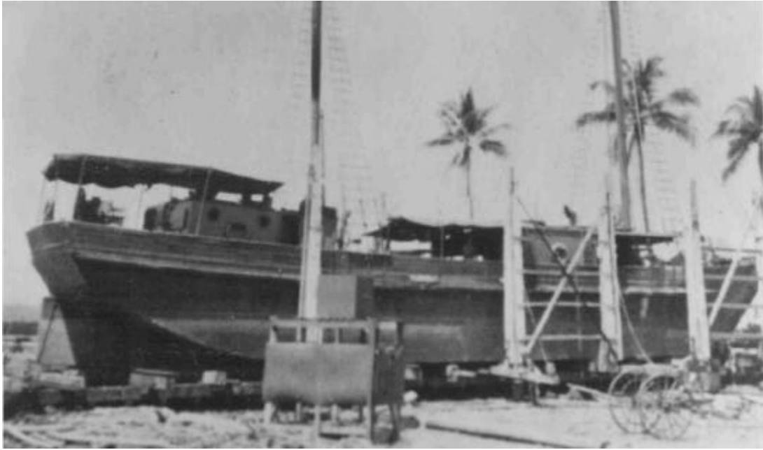
“Betty Joan” undergoing anti fouling to her hull while on the Navy Slip at HMAS “Tadova”, Milne Bay, October 1945. (Alf Wilson)
