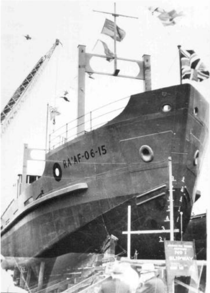
06.15, a steel constructed vessel, 120 foot long, was one of the newly designed Cargo Boats.
