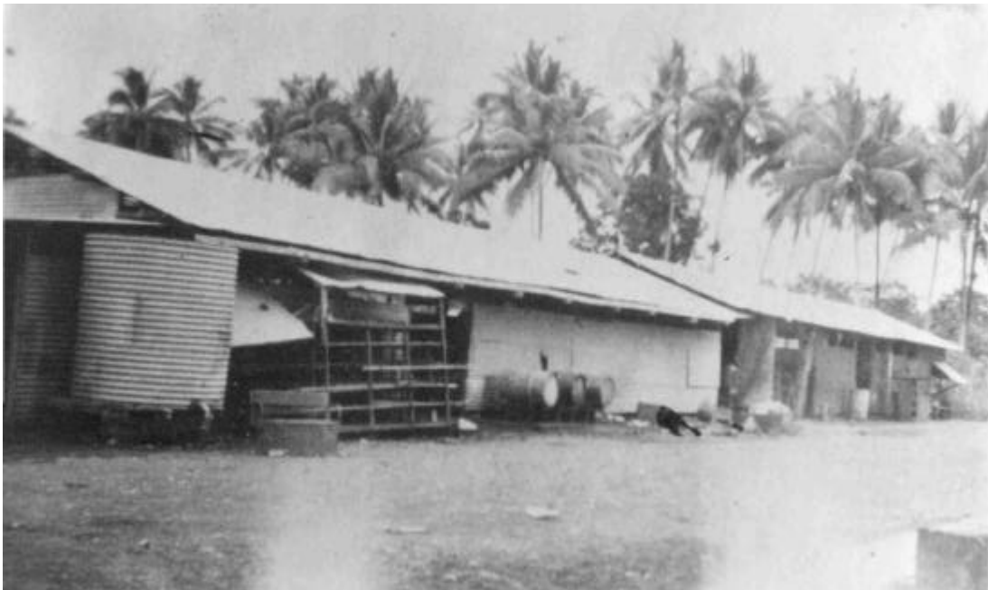
A section of the Marine Section Workshops where major engine maintenance and modifications were carried out. (Alf Wilson)
