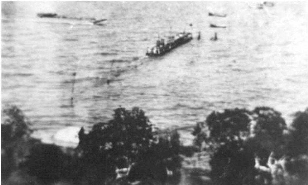
The West Bay jetty was another asset built by the Marine Section, & at high tide part of it is under water. Off shore the boats are on moorings. (N.Greaves)
